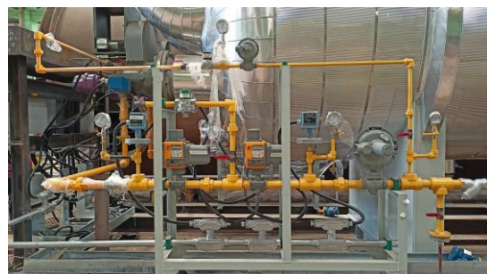
Integrated Skid with Control Panel for Gas Burner Valve Train
